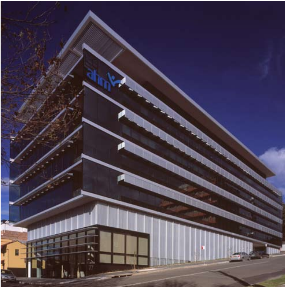
Left Building exterior Right Lobby
